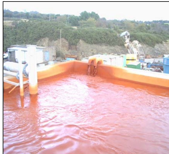
Figure 4. Stage I reactor
